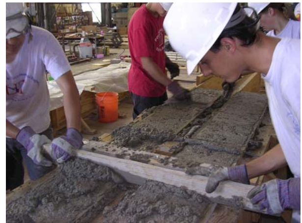
(b) Screeding Concrete Surface
