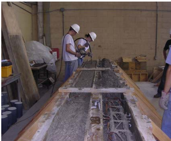
(a) Vibrating Concrete
