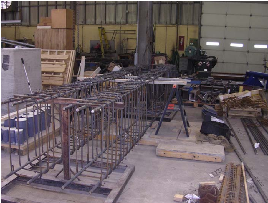
Figure 2.7: Fabricated Rebar Cages
